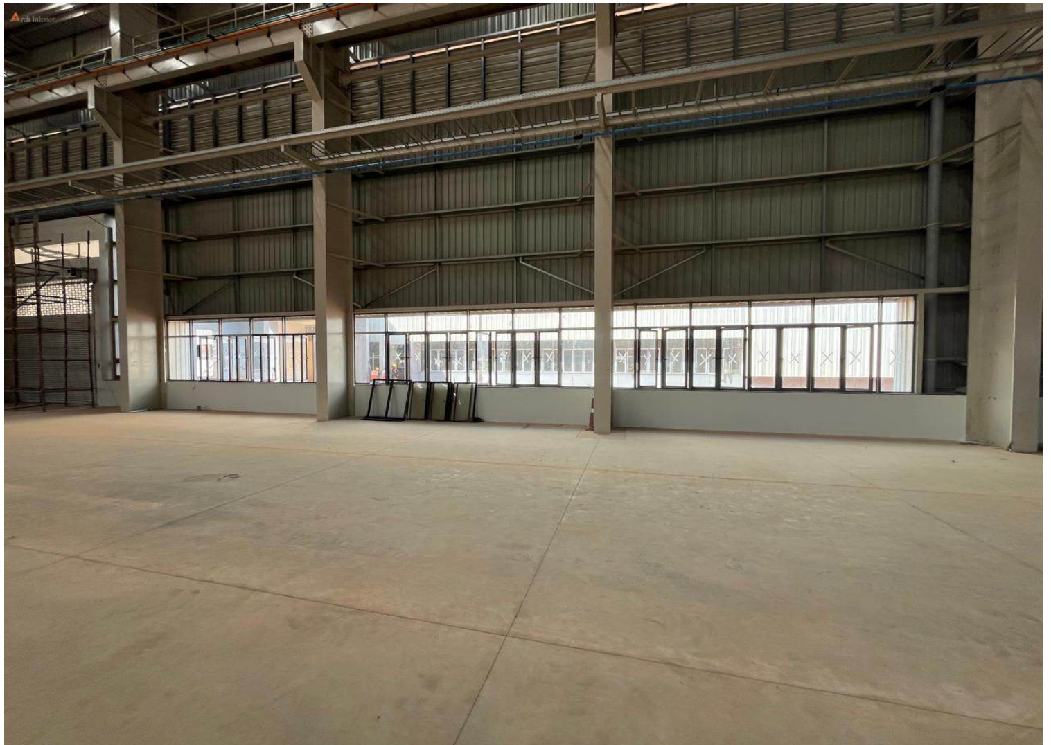
COMPLETED SITE IMAGES
